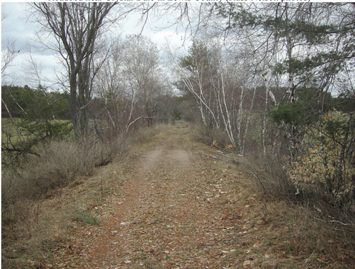
Roadbed near Crystal Dale in Lewis County (Russ Nelson photos)
